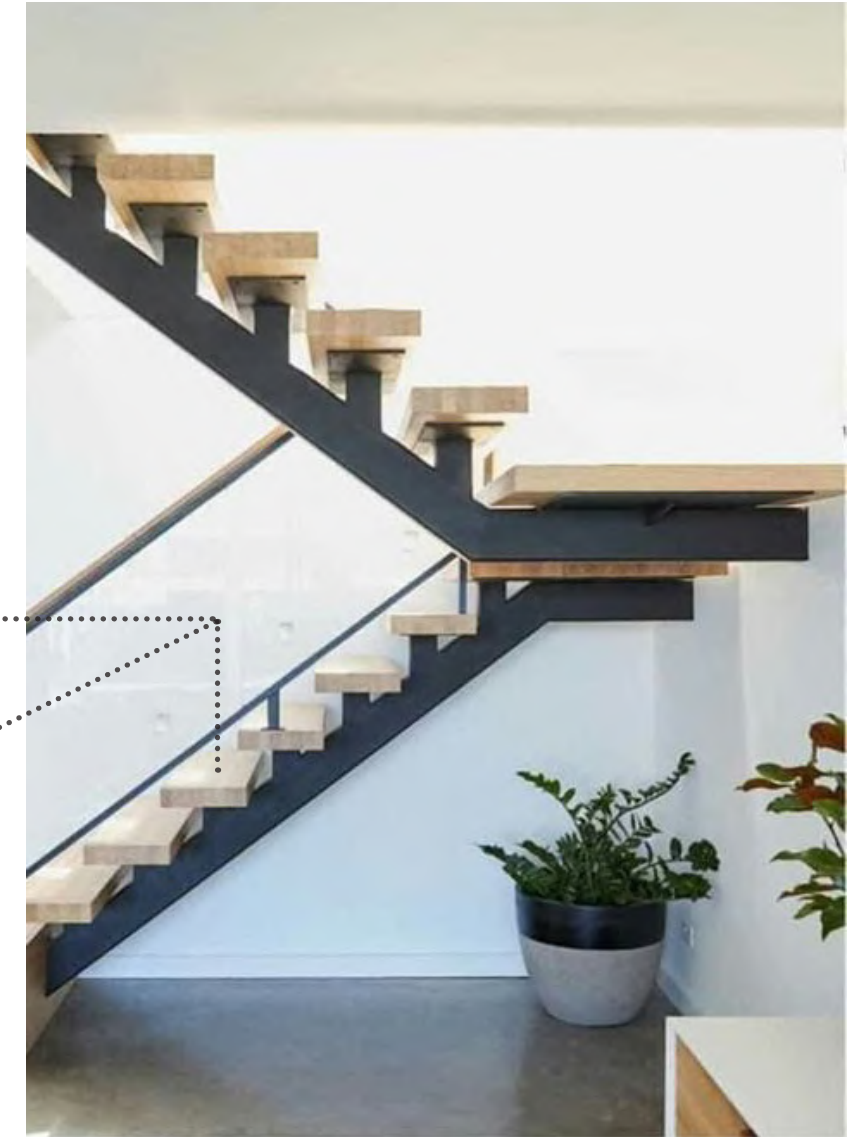
OPEN TREAD AND GLASS RAILING TO START ON FIRST LEVEL AND STOP AT LANDING. GLASS RAILING TO OCCUR ONCE AGAIN AT 2ND LEVEL LANDING.
