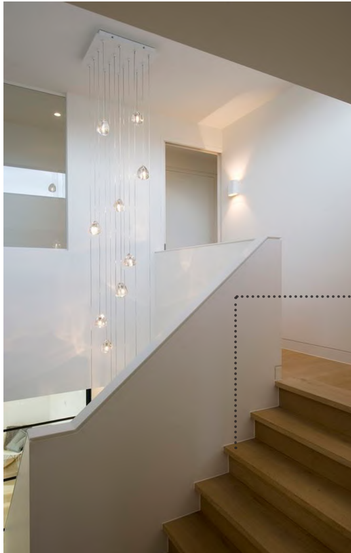
CLOSED TREAD AND DRYWALL RAILING TO START AT LANDING AND CONTINUE UNTIL 2ND LEVEL
